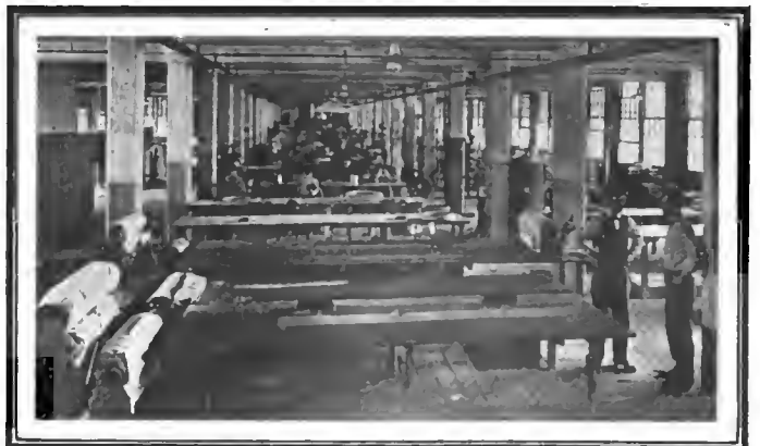
Repair room of the Goodyear Tire & Rubber Company, Akron, O.
